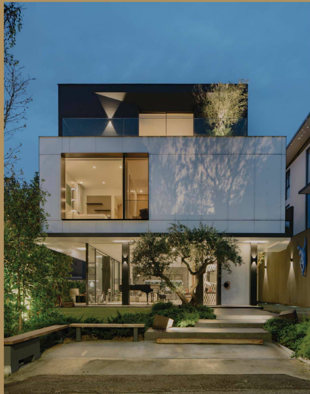
A GENEROUS GARDEN AND SEATING FOR PASSERS-BY ARE CREATED BY EXCLUDING A CAR PORCH.
