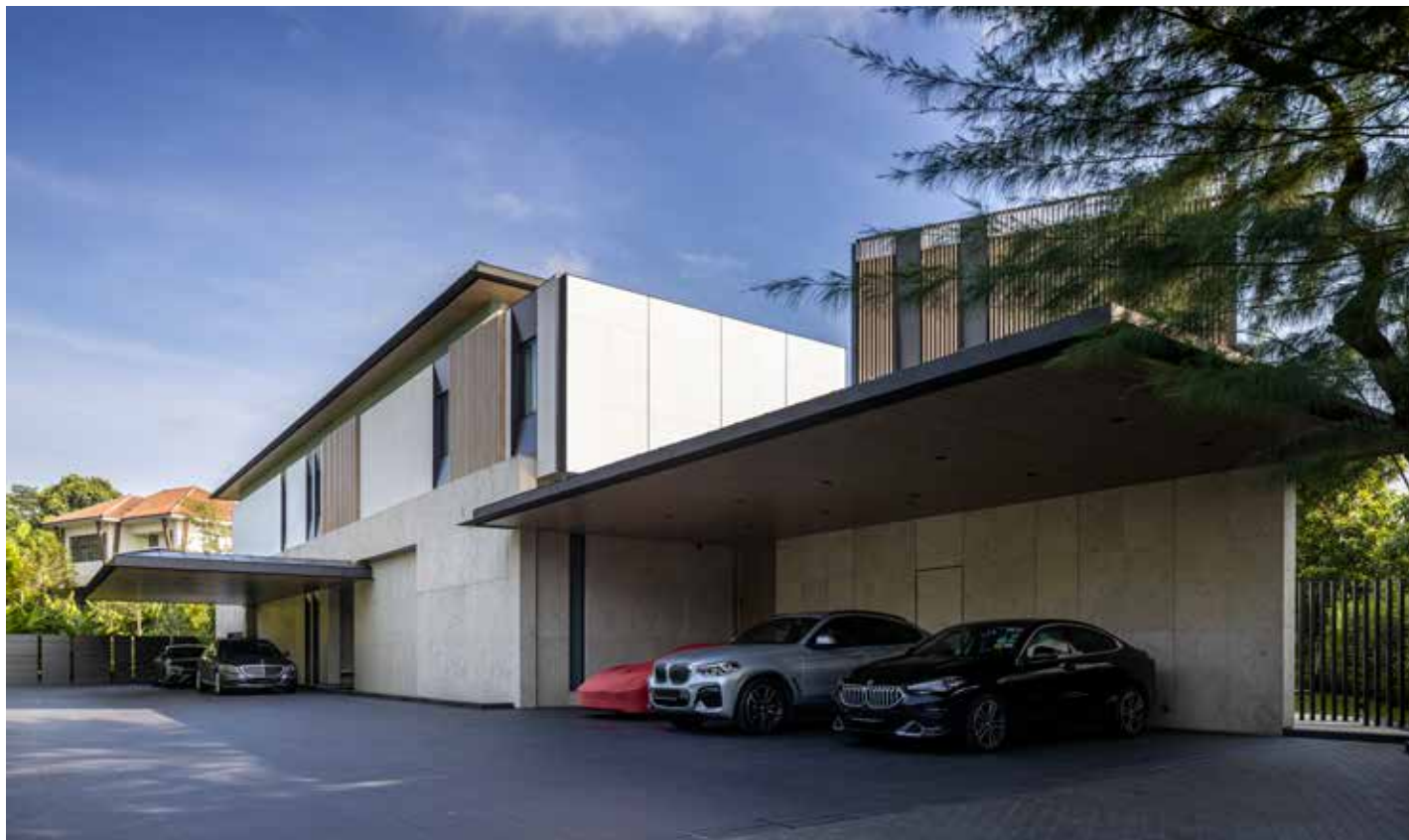
The majority of the façade showcases a honed finish for a smooth and refined appearance.
