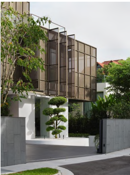
ABOVE The Metallicus features aluminium screens that are among its most distinctive features
